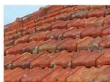
Existing Roofing (RF.EX.01) Terracotta/Clay Tile
